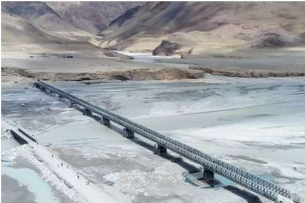
Figure 7: Areal view of the Strategy Structure with automated crack detector
