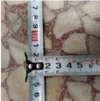
Figure 8:South left corner
