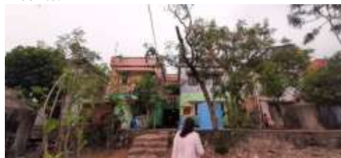
Two storied Tsunami rehabilitation houses
