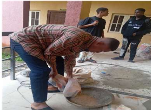
Plate 6: Batching of fine aggregate
