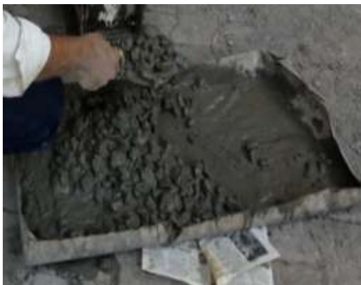
Fig.: Mixing of concrete by hand in pan
