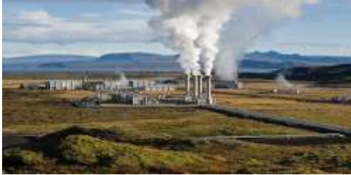
Geothermal power plant
