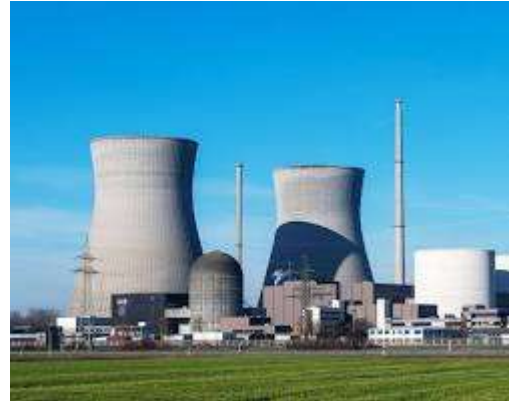
Nuclear power plant
