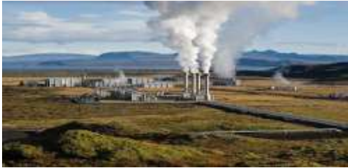
Geothermal power plant
