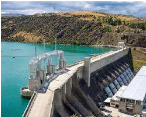
Hydroelectric power plant
