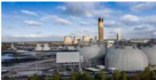
Biomass power plant
