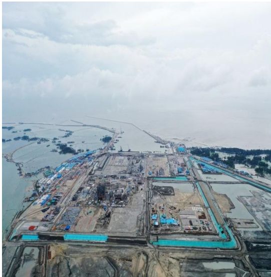
Figure5: Matarbari coal power under construction plant
