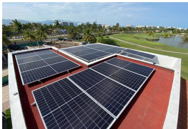
Figure 2. Installation of Jinko Solar Tiger Pro type SP on the roof with the required spacing
