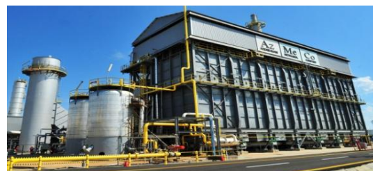
Figure 1. General view of the methanol plant built by the AzMeCo company in the Gobustan region
