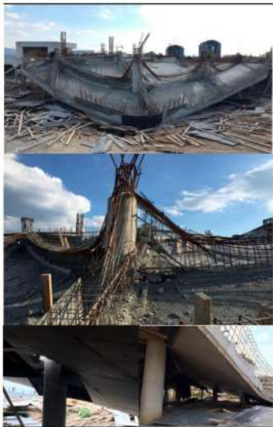
Figure 9: Images of the collapsed part of the building due to the punching effect[1]
