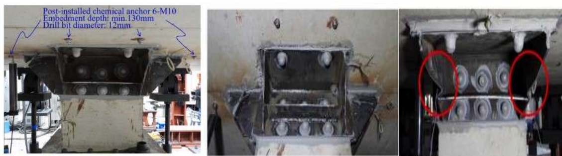
Figure 8: Attached column head steel plate to slab (red circles indicate buckling) [2]
