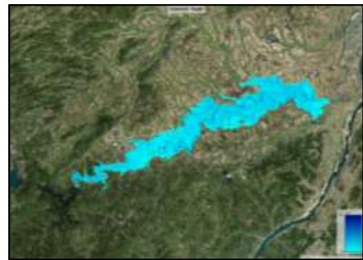
Dam failure 20 h
