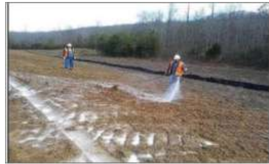
Fig. 1: Mixing Stabilizer to Soil
