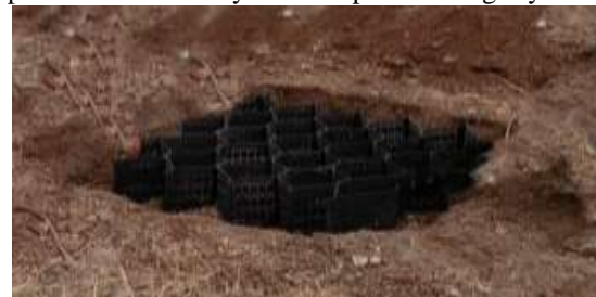
FIG. 3 LAYING OF GEOCELL
