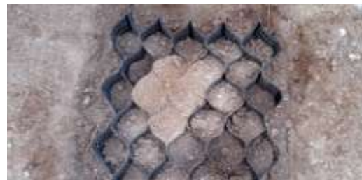
FIG. 4 PLACING OF INFILL MATERIAL
