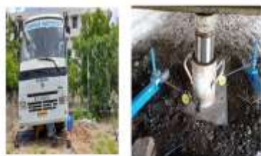
FIG.8 SET-UP OF PLATE LOAD
