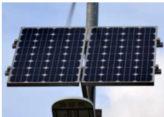
Fig-5: A solar board that is comprised of octagonal monocrystalline silicon cells.
