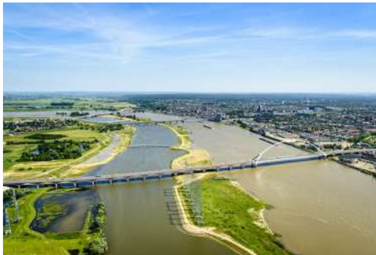
Room for the River Programme, Netherlands
